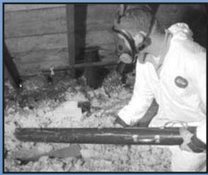
Removal of insulation contaminated with bat feces
