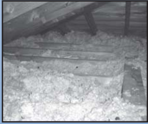
Trampled insulation
