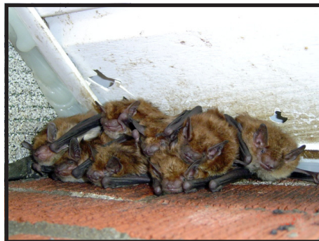
Bats roosting in corner of attic
